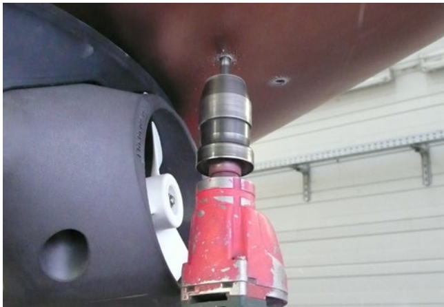
Fig. 19: mounting bolts drilling
