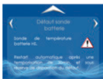
Description of faults and fault clearing conditions
